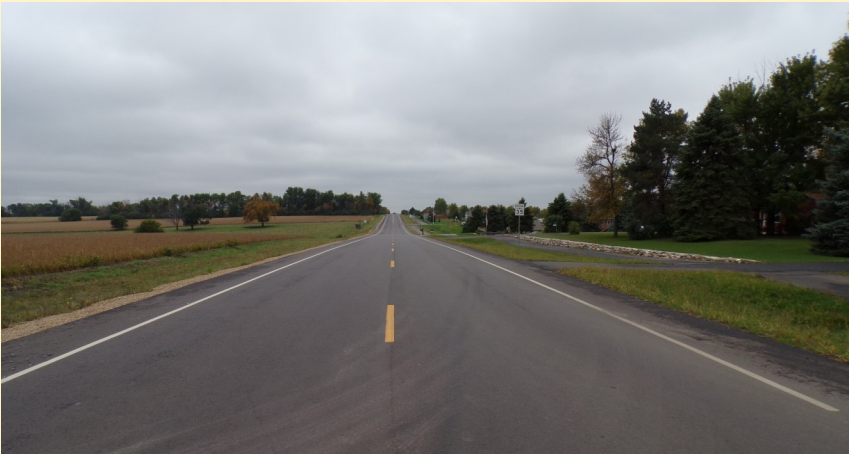
County Highway 149 reconstruction in Hartford, SD looking south
